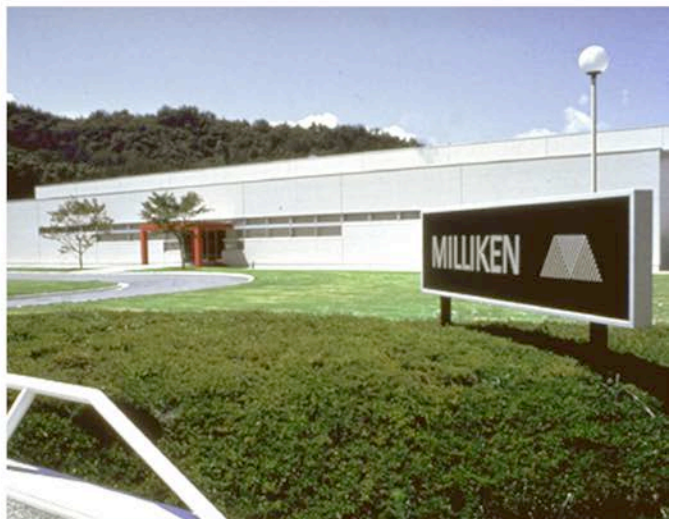
Milliken Design Center and Production/Distribution Facility Program Management & Design Consultant
